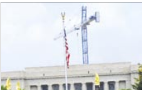
Rex Freeman operates the tower crane at the Marion County Library.
