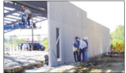
Construction begins on the new Indianapolis office building
