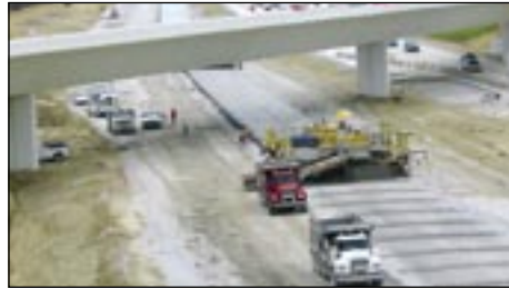
Berns Construction working on I-70.
