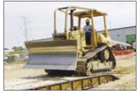
Roland Neal runs a bulldozer at the new Indianapolis building site.
