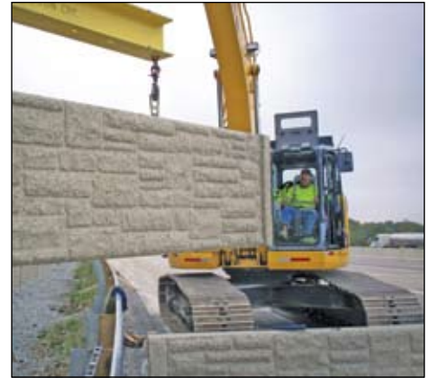
Anthony "AJ" Poulton setting the wall on 465 for Kokosing Construction Co..
