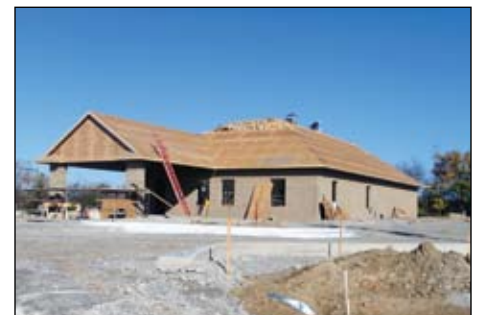
Fort Wayne union hall gets its roof.
