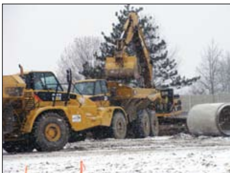
Fox Contractors doing the sewer work at the new Parkview North.
