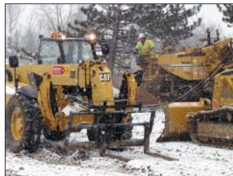
Fox Contractors and Shambaugh & Sons working at Parkview North.
