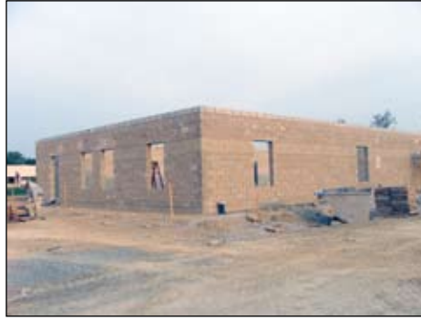
And the walls go up on the Fort Wayne union hall.
