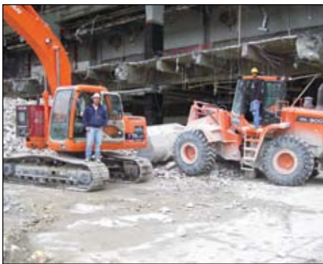
Wade Sparks and Brian Stidd at the RCA Dome demolition project.
