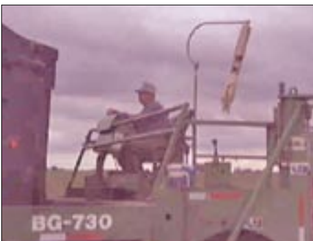
Carl Ross on SR 124 running the widener for E & B Paving.
