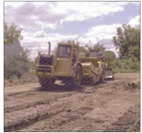
New apprentice, Brandon Leas, gets a load on 621F scraper.
