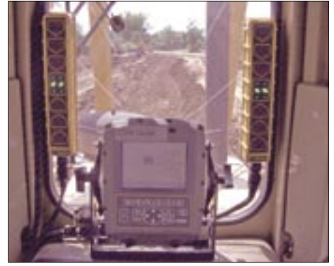
The Training Site is keeping up with the times with a D5M Dozer full loaded with a GPS System.
