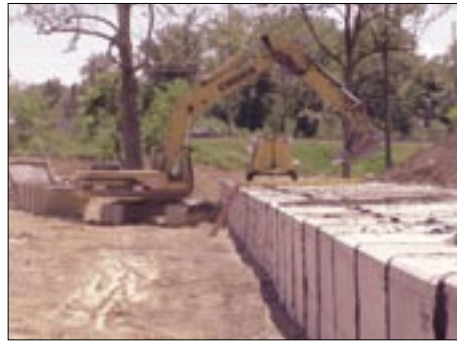
Wes Kleiber working for Crider & Crider on a box culvert.
