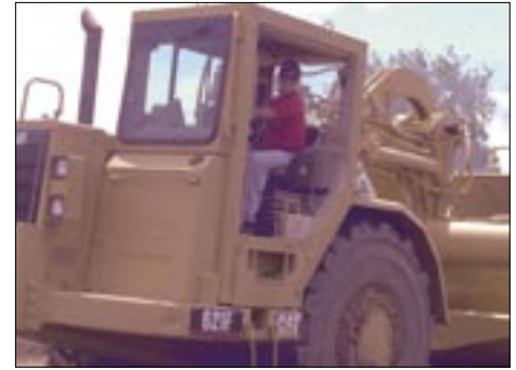
New apprentice, Brandon Leas, checks his grade stakes as he cuts.
