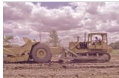
Robert Pyles, a new apprentice, pushes scraper for a full load.
