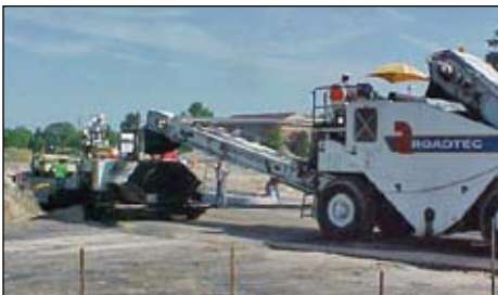
Eric James runs the paver while James Leach is on the shuttle buggy. Leonard Allred is behind rolling the asphalt.
