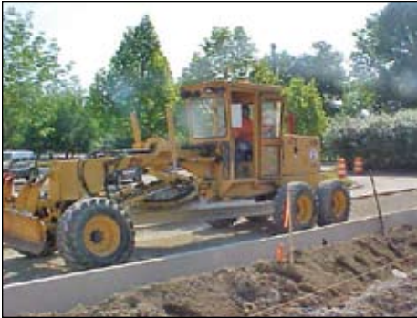
Randy Bell operating a grader on McKinley Ave. at Ball State.
