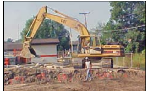
Ned Bynum at the Ossian WWTP for Thieneman Construction.
