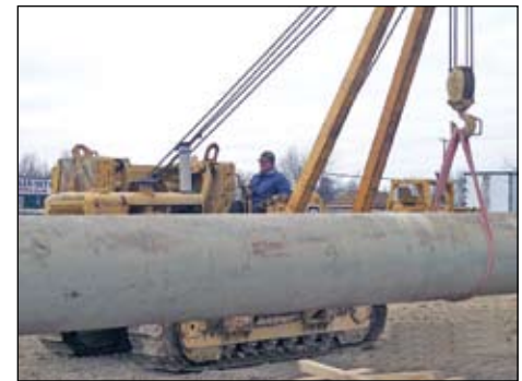
Gary Johnson running the sideboom at the training site.
