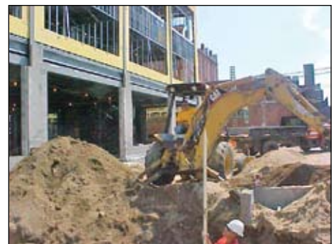
Troy Watters at Gale Tschuor job on Walnut Street in Muncie.
