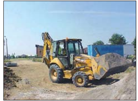
Dave Toland working for Fox Contractors on SR 1 in Ossian.
