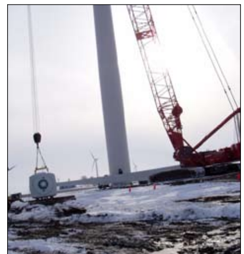
Bill Parson setting the turbine section of the windmill.
