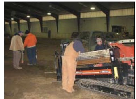
Apprentice Ray Turner operating the directional bore machine.
