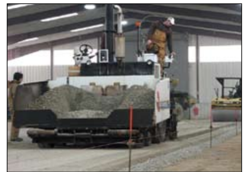
Apprentice David Sams operating the Road Tech Paver.
