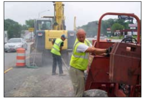
Jeff Bercot working on the Jefferson Blvd. project.
