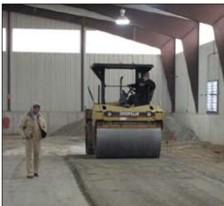
Brian Bramer observes Micah Rawls rolling patterns during asphalt class.
