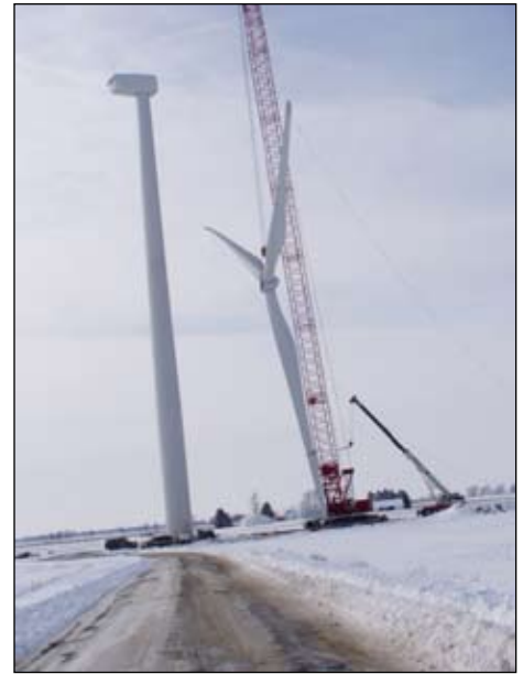
Ron Pell setting the turbine blades at the Windmill Farm.
